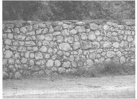
Figure 14 – Stone fence made of pebbles in Palaionastiro village
