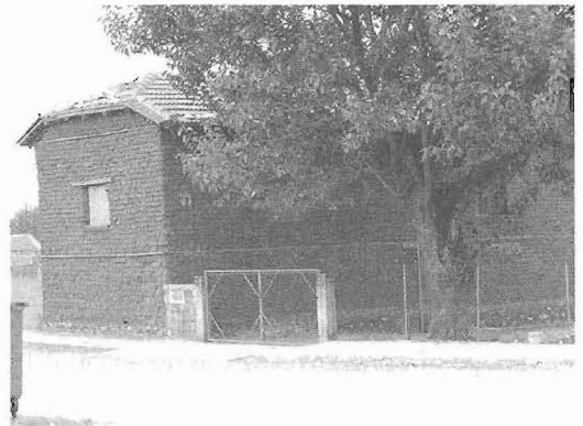
Figure 11 – Stable made of mud-bricks
