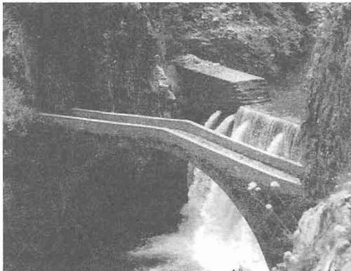
Figure 23 – The reconstructed old bridge at Paleokaria village
