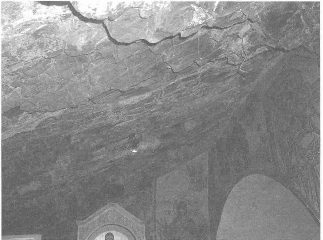
Figure 7 - Ceiling view of section B. Unsupported Section. The north western corner of the section, appearing the rock falls, is clearly presented
