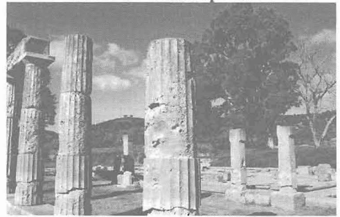
Figure 15 - Different degree of decay on column pieces
