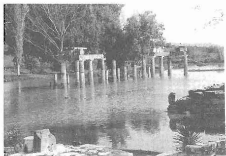
Figure 27 - Brauron monument (26/11/2005) Erasinos flooded after strong rainfalls
