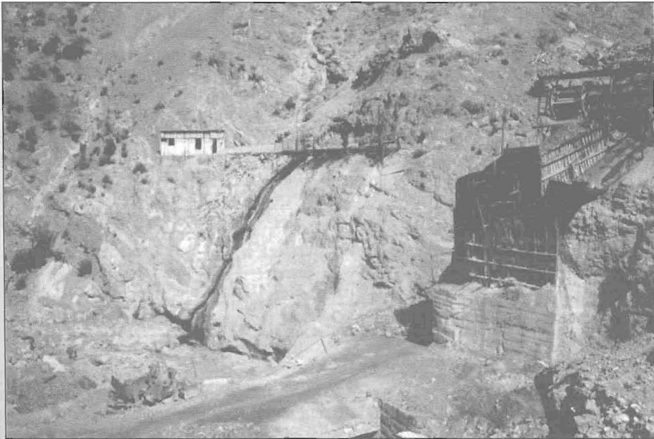
Figure 2 - Acid waters flowing from the Spaci Repsi Mine area
