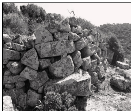
Figure 2: Examples of horizontal displacement in the walls of nuraghs from northern Sardinia (Sos Tittinosos, Pattada)
