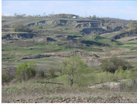
Photo 6: Successive detachment scarps on the waste dump placed on the slope, at Seciurle
