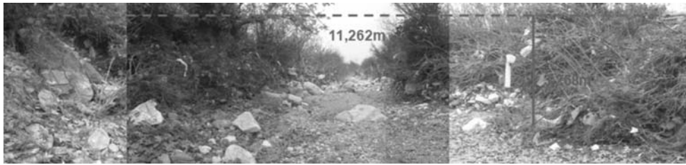
Fig. 10: Photo of Xerias stream. No erosion has been observed.
