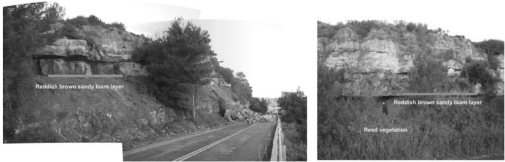
Fig. 7. The layer of reddish-brown sandy loam is slowly washed out by the percolating water from the overlying limestone (note the beginning of undercutting). The water favors thick reed vegetation. It is a matter of time this slow process to undercut the limestone causing a rockfall in this place in the future.
