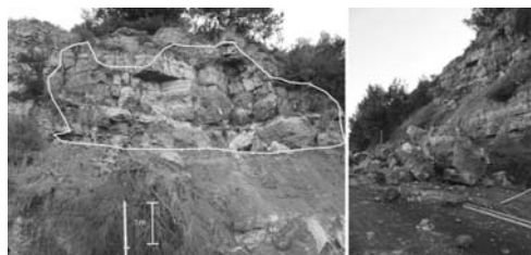
Fig. 4: Source area of the December 21, 2009 rock falls.
