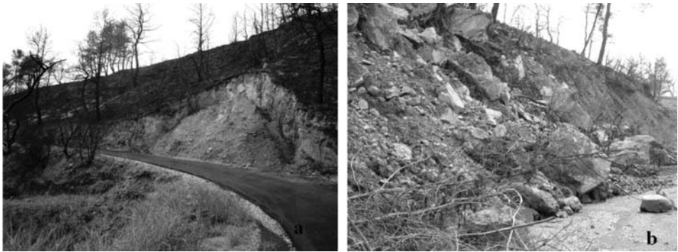
Fig. 5: Significant Landslide phenomena in (a) the road of Koumouthekla – Makistos and (b) outside the Koumouthekla village.
