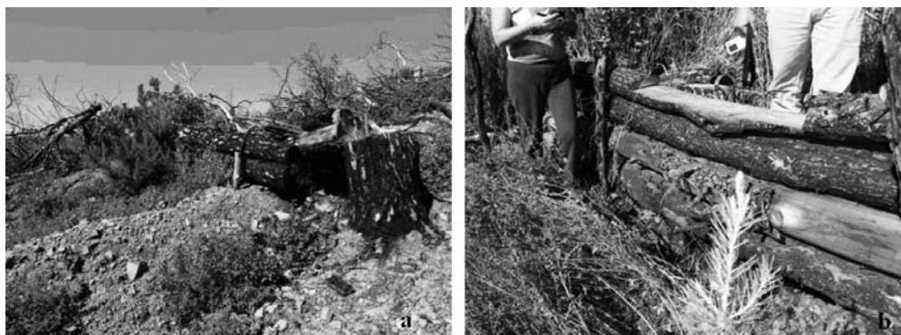
Fig. 9: Failure of log-barrier (a), and effective implementation (b).
