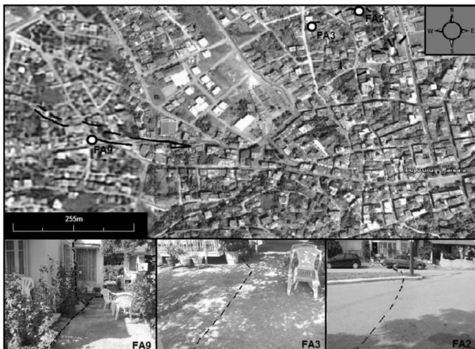
Fig. 4: Satellite pictures (from Google Earth) pointing the location of the surface raptures along Farsala town. Pictures FA2, FA3 and FA9 show roads and buildings damaged by the surface raptures.
