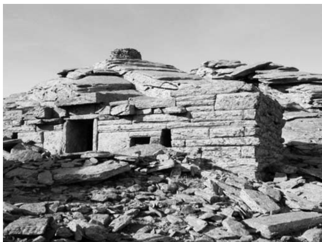
Fig. 1: The Mt. Óchi Drakóspito: External view.
