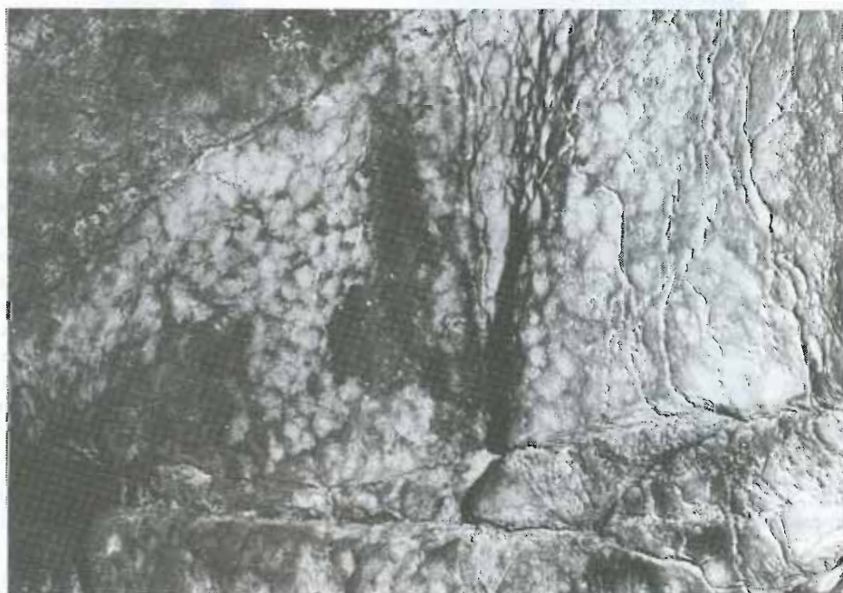
Fig. 5 Scalloping on the wall on the top of the shaft of SH. The average size of scallops in 1 inch.
