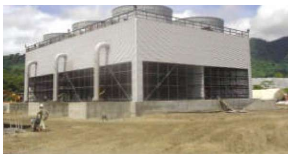
Lihir Power Station.
