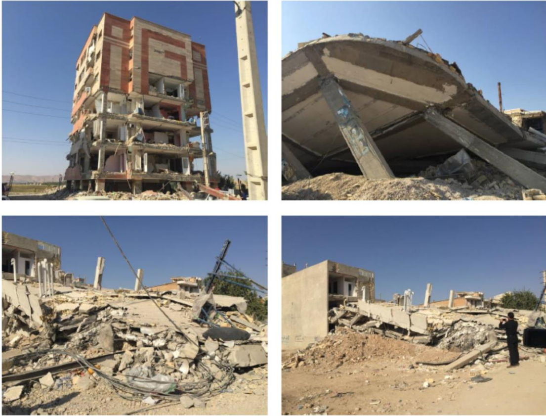
Figure 5.2 Building failures in Sarpol-e Zahab city. Images are from Zare et al. (2017) earthquake report.
