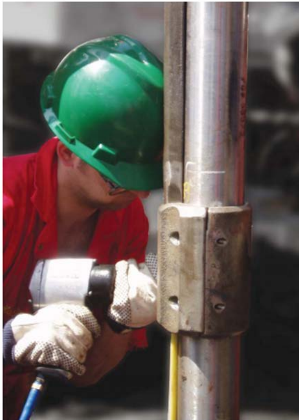
Fig.4.32 Installing a control line protection plate (Bellarby, 2009).
