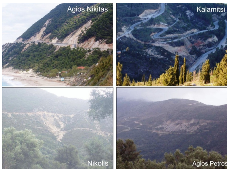
Figure 3: a) Rockfalls in the provincial network for Agios Nikitas (the longest landslide in Lefkada), b) Flat slides on the rocky slope to the road network near Kalamitsi, c) Landslide near Nikolis village, d) Rockfalls in the provincial network for Agios Petros in Lefkada island
