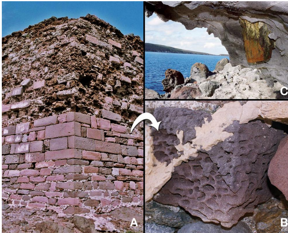
Fig. 5. A-B: tafoni formations from the Sigri Castle walls, figure C: a petrified trunk and tafoni on the same formation. A unique image of Geoparks comprehensive perspective.
