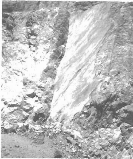
Figure 9a: The E-W normal fault zone affecting the preneogene limestones to the west of Kechries peninsula
