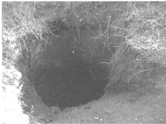
Figure 8: Collapse of the filling of a karstic chimney crossed by Dodoni Tunnel. The collapse outcropped on the surface about 100 m. over the tunnel.
