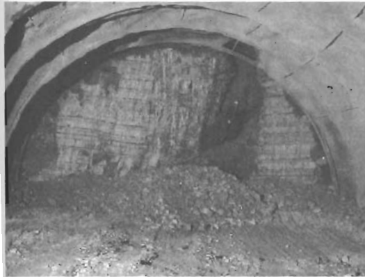
Figure 7: Typical appearance of a small karstic void partially filled with clay and silt; Dodoni tunnel, northwestern Greece, 2000.
