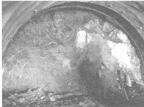
Figure 1 - Medium to poor quality gneiss and good quality marble
