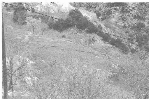
Figure 2 - Rotational slides affecting the terraces
