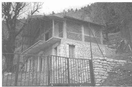
Figure 3 – Reconstruction and extension of an old house
