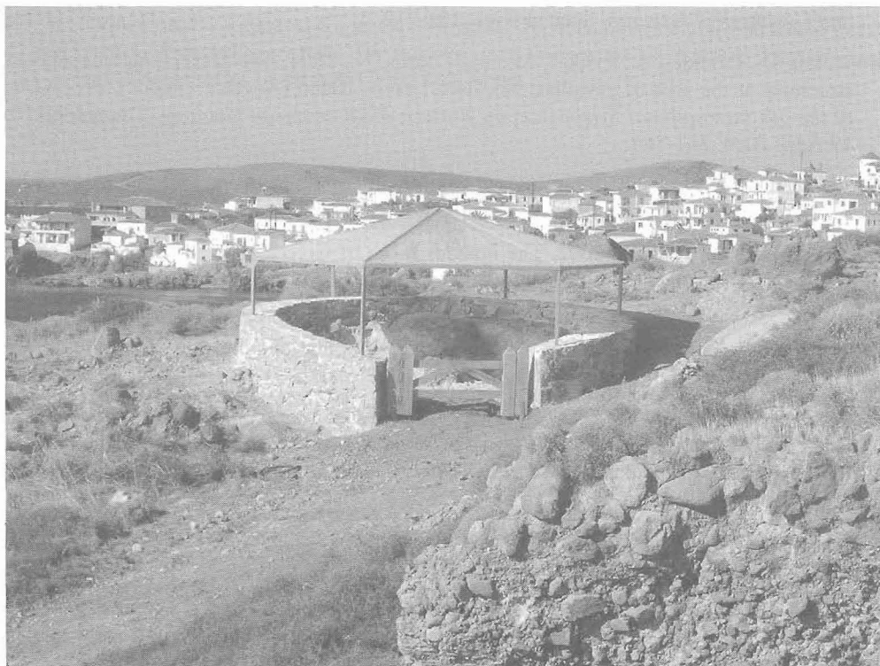
Figure 8 – Protective shelter in the Plaka park for a standing petrified tree trunk excavated within the coarse conglomerates layer of the Sigri pyroclastics formation
