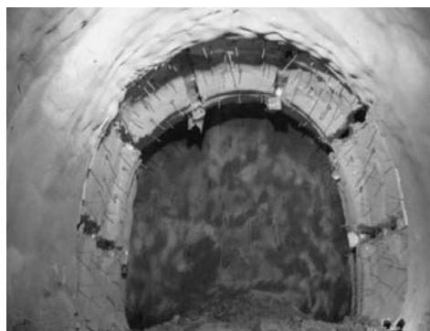
Fig. 9: Yielding cross section Y45.g – primary support.
