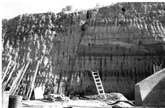
Photo 2: Northern portal of tunnel SA (left branch). The Pliopleistocene sediments are characterized by almost horizontal dipping. The Lower unit, grayish blue in color, is progressively changing, through the transitional zone, into the light gray Upper unit. In the centre of the Figure a normal fault is presented, that has substantially change the previous sequence and thus the slope (in the left hand site of the figure) is only occupied by sediments of the Upper unit.
