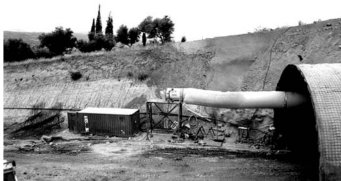
Photo 2: South part of Girokomion tunnel ( \Sigma 2 ), right branch. The Diluvial conglomerates cover with unconformity the Upper Geotechnical unit.
