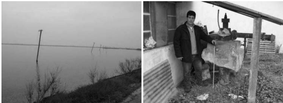
Fig. 2: (Left) Submerged remnants of the old electricity network constructed along the side of a road, SW of Kalochori, in 1975. (Right) Emerged well's pipes at a 100 m deep well located in the Institute of Wheat Cultivation (SW of Kalochori). The pipes have been extracted 0.8 m over the ground surface. The photos were taken in 2008.
