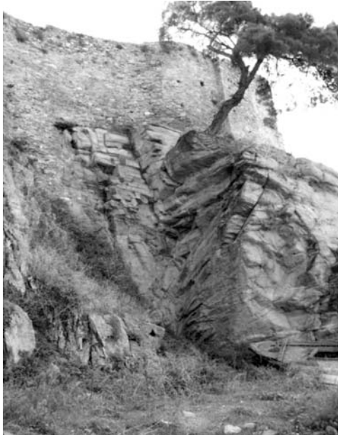
Fig. 2: Location P1. A fault intersects the slope forming a huge rock wedge and a wide fractured zone. The Wall fills the gap between the two sections of the fault.
