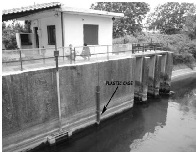
Fig. 2: STATION 1 was put at the beginning of irrigation network of Nestos river basin, in a floodgate room in WAC. A plastic case was plunged into WAC and the sensors were put inside the case to be protected.
