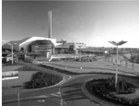
Fig. 4: WTR facility in Brescia.
