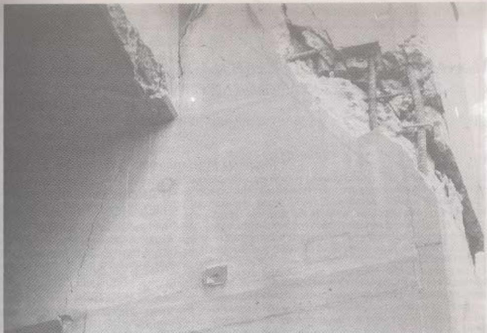
Fig. 8: Detail of the damage produced in the Nimitz Freeway.
