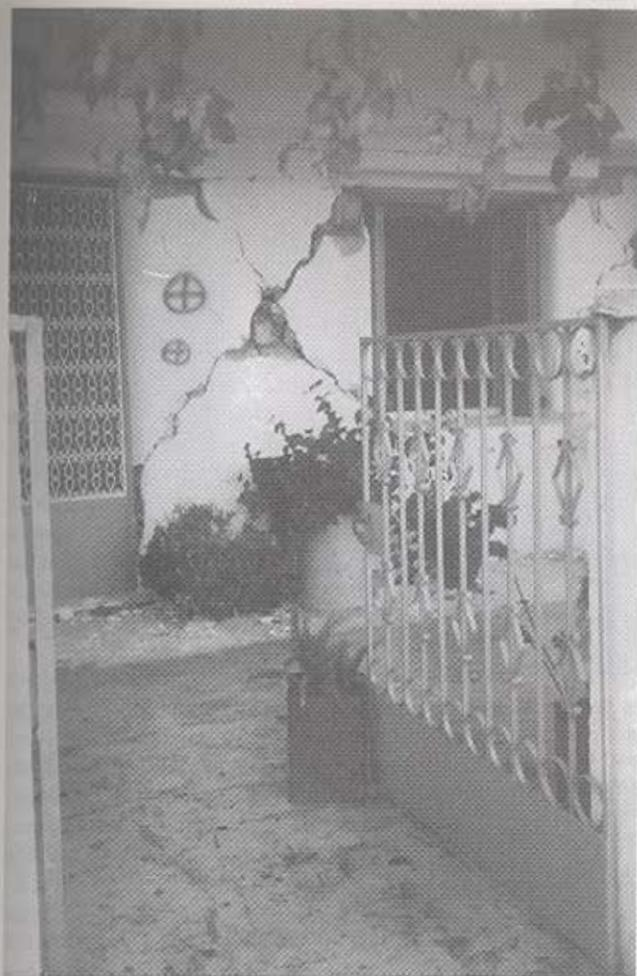
Fig. 2: Typical damage in reinforced concrete house in Kastro.
