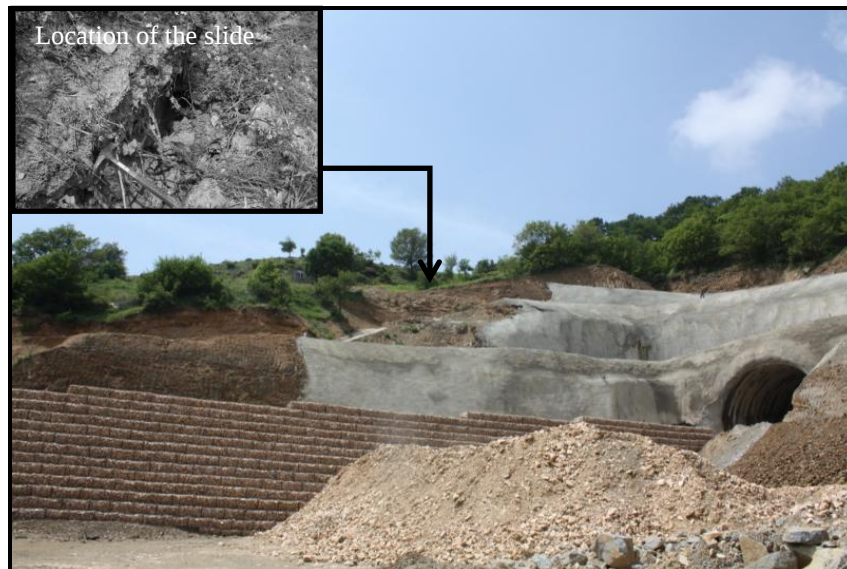
Figure 1 - View of the entrance portal of Nymfea tunnel. The gabion wall is used here for the stabilization of the whole slope. The slide occurred above the gabion wall.
