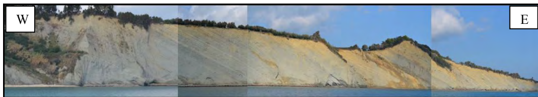
Figure 3 - Panoramic view of Section three.
