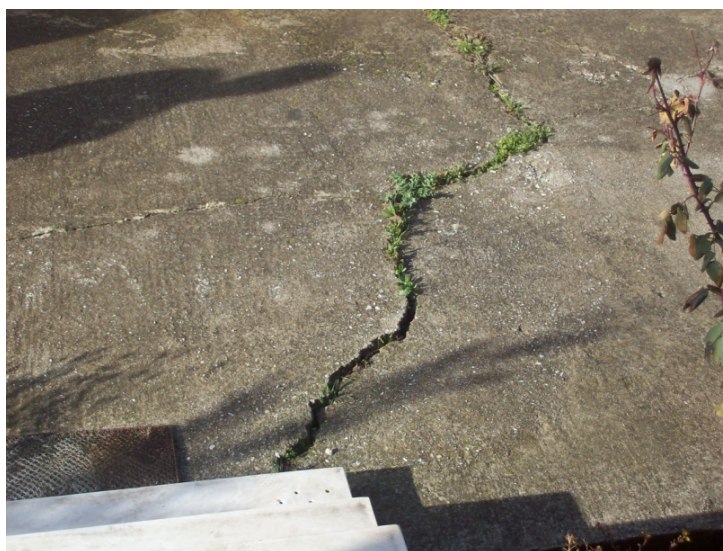
Figure (1.4) : Image of the surface fissures in Anargyroi village (after Soulios, 2009 ).
