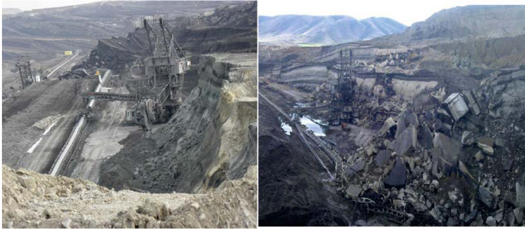
Figure (6.1) : The 14 th January of 2014 landslide in the mine open-pit.
