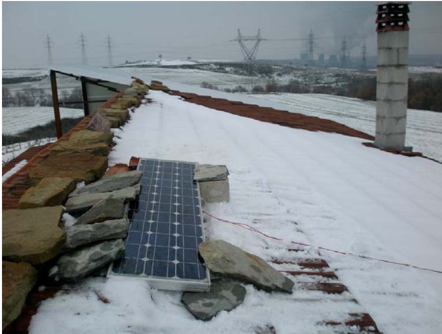
Figure (4.4) Solar panel for supplying the seismological station codenamed ANAN (Tsapanos et al., 2011).
