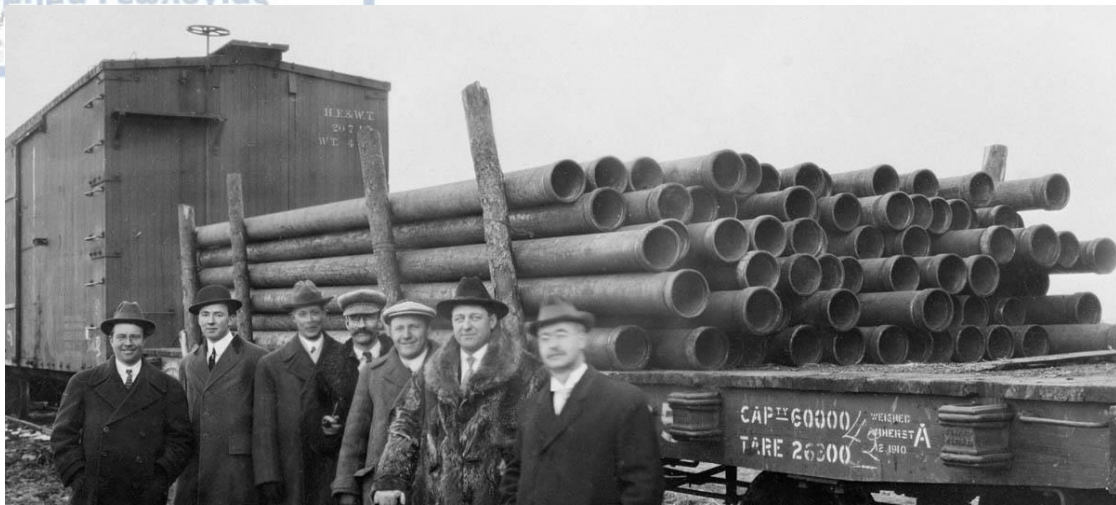
Image 1: Construction of natural gas pipeline by Northwestern Utilities Company Limited in Canada, 1923
