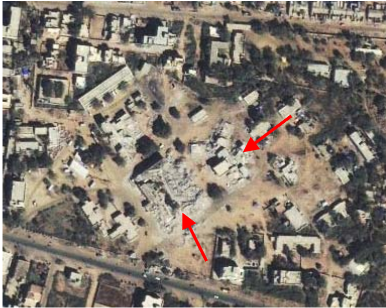
Fig.7: In the middle of the Ikonos image are clearly two collapsed buildings.
