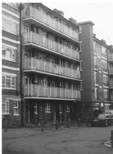
Photo 5. Council housing, Shadwell, 2001.
