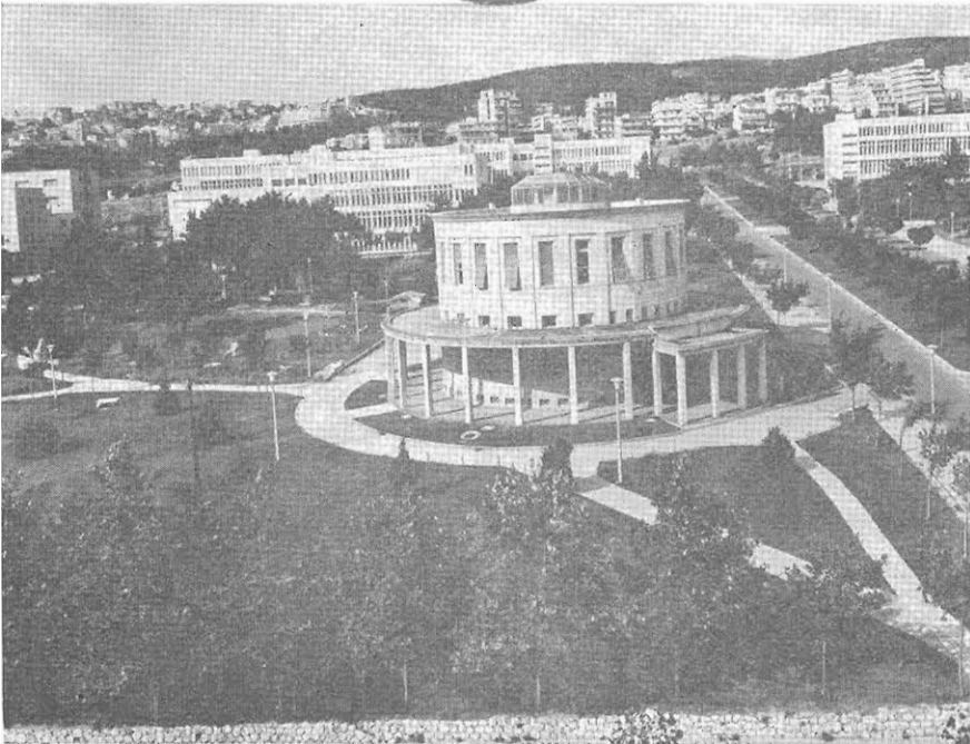
Fig. II. Second period: January 1958 - to date. New building of the Institute of Meteorology and Climatology (Elevation 44.65 m (M.S.L.).
